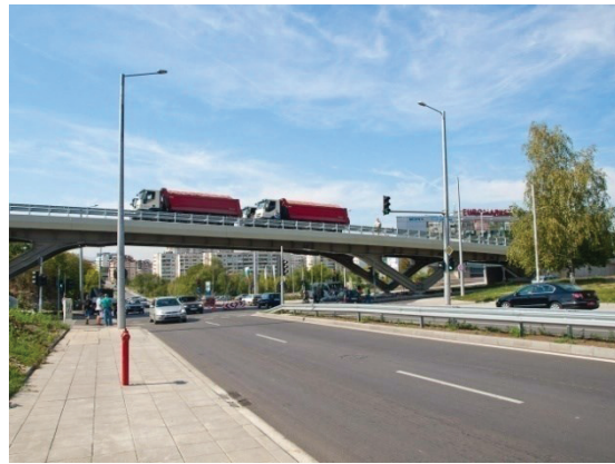
c) Steel road bridge
