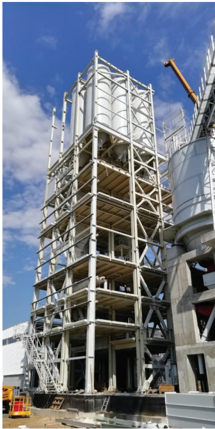
a) High-rise industrial steel structure with CBFs
