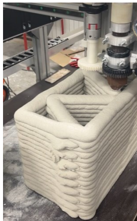
Figure 5. The process of 3DCP of individual segments
