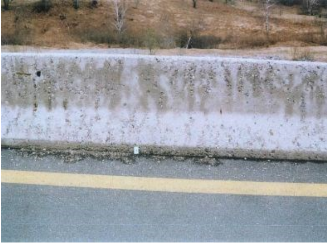
Figure 1. Safety barrier built of traditional concrete with NRA
