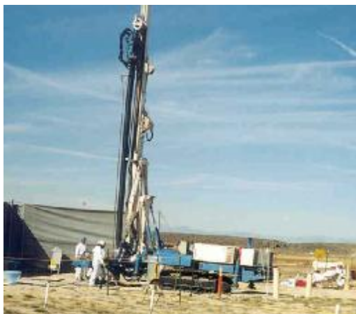
Slika 8. Jet Grout Drill
