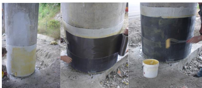
Figure 4.3. Confinement strengthening (Di Ludovico M. [21])
