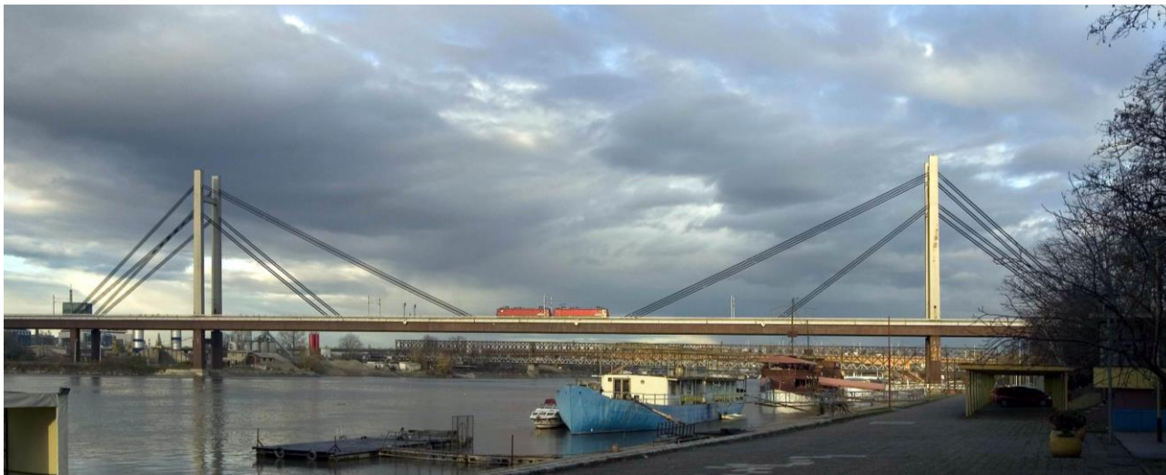
Slika 1. Železnički most preko Save u Beogradu (autori – projektanti: Nikola Hajdin i Ljubomir Jevtović) Figure 1. Railway Bridge over the Sava River in Belgrade (authors-designers: Nikola Hajdin and Ljubomir Jevtović)
