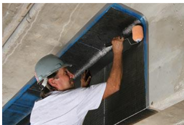
Figure 4.4. FRP strengthening of a beam (CNR-DT, [8])
