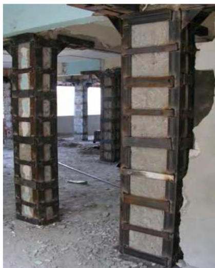
Fig.2.5. Steel jacketing applied to RC columns (M.N.Fardis, [12])
