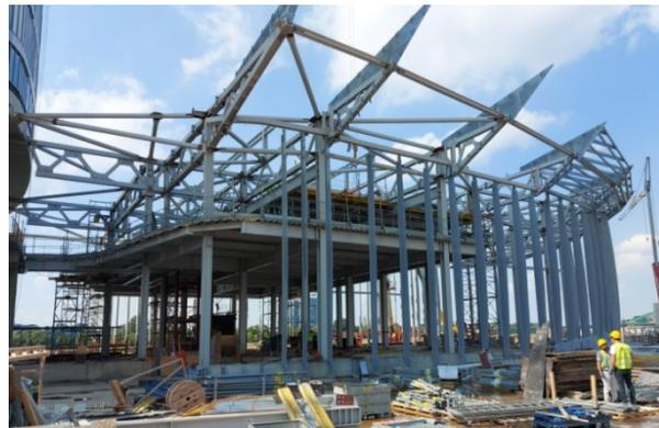
Figure 9. Podium Roof Steel Structure
