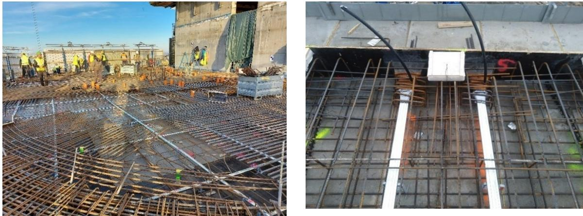
Figure 16. Reinforcement and PT works in progress
