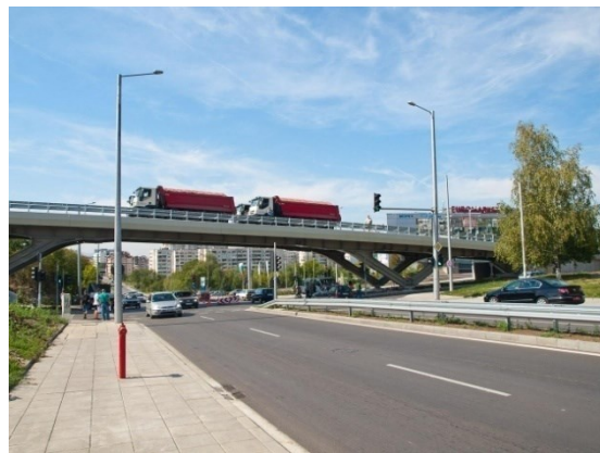
c) Steel road bridge
