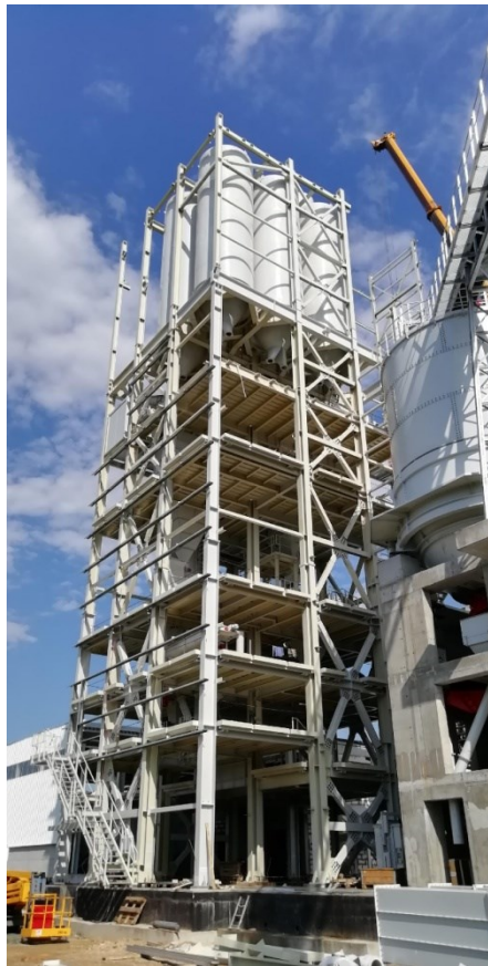
a) High-rise industrial steel structure with CBFs
