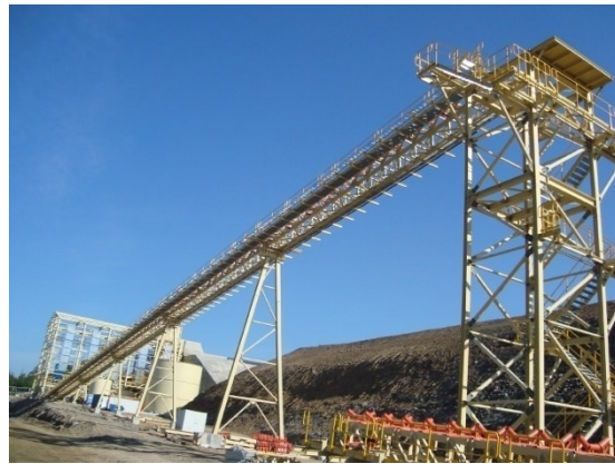
b) Belt conveyer with high-rise trestle
