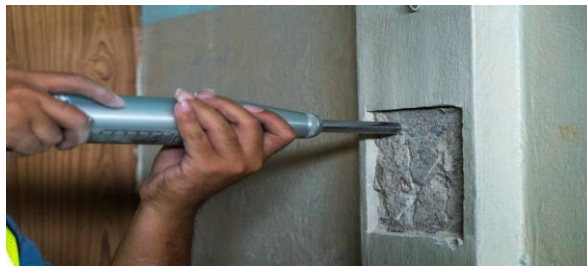
Fig. 2. Schmidt rebound hammer
