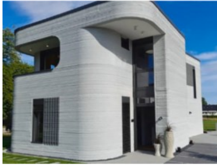
Figure 1. Two-story Beckum house [13]
