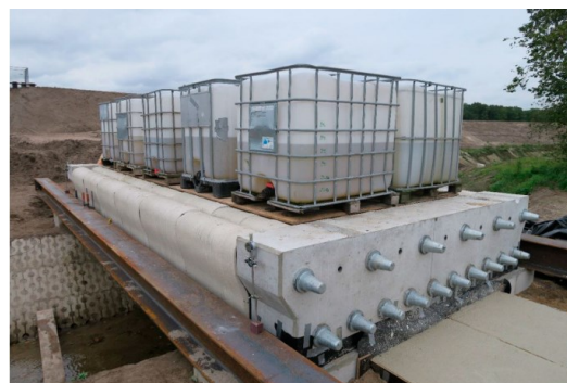
Figure 4. In situ testing of the bridge with water-filled containers [23]
