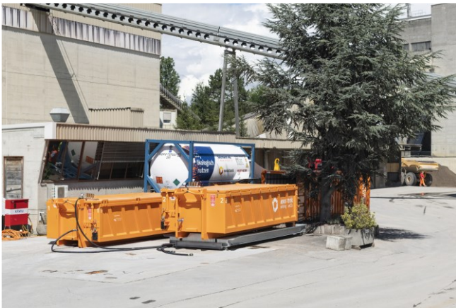
Figure 6. Industrial mineral carbonation plant (two reactor containers, CO 2 storage tank and centre for the process control) [90]
