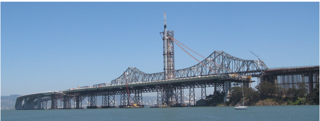
Figure 13. New East Bay Bridge under construction (2011)
