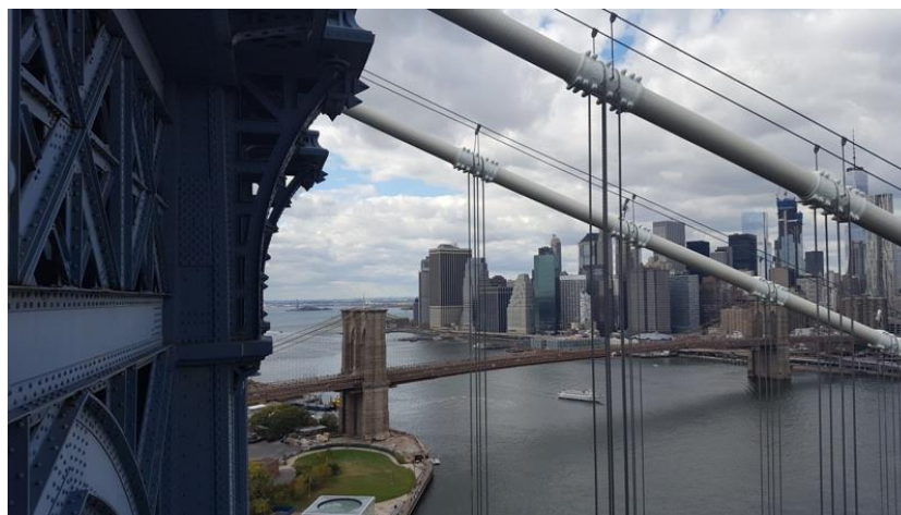
Photo 3-BY. Suspenders in Manhattan Bridge
