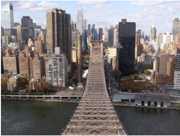
Photo 2-BY. The Queensboro Bridge
