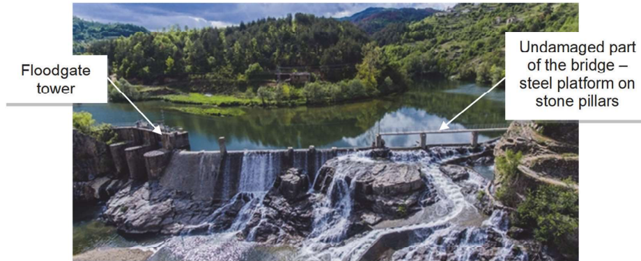
Figure 2. Existing situation after accident. The destroyed part of the pedestrian bridge
