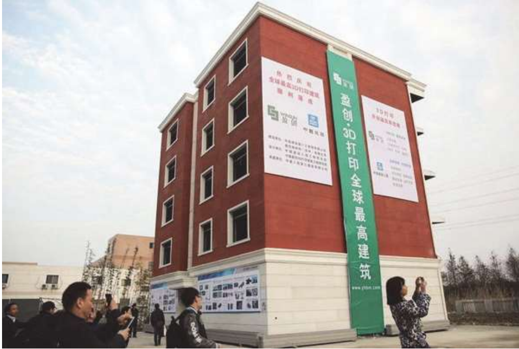
Slika 2. Petospratni stambeni kompleks kineske kompanije WinSun, 2015 (1100m 2 ) [14] Figure 2. A five-story residential complex by Chinese company WinSun, 2015 (1100m 2 ) [14]
